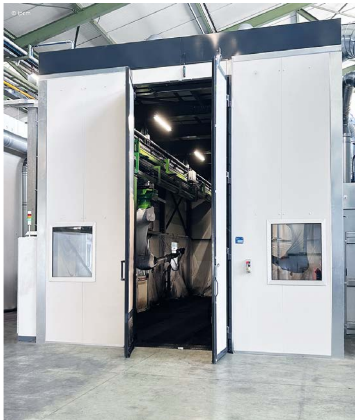
The outside of the UV top coat application booth.
